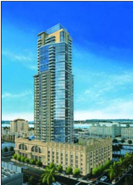
Bosa maintained the exterior of the historic SDG&E building while creating a new tower inside the shell of the existing structure.
